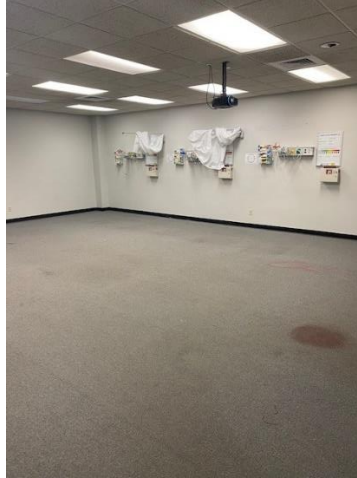
Nursing lab getting ready for new flooring
